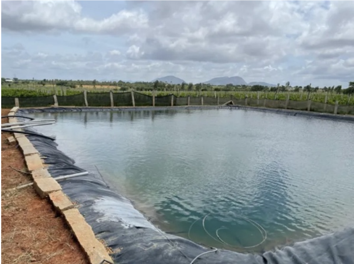
Rain water harvesting pond
