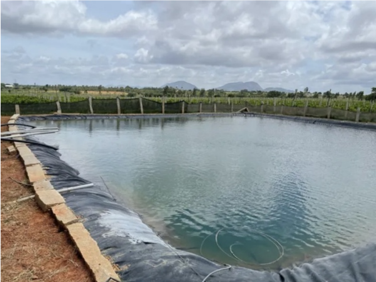
Rain water harvesting pond
